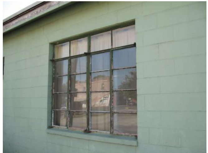
Metal casement windows were commonly used in commercial and industrial buildings in the late 19th and early 20th centuries. (1433 W. Main Street)
