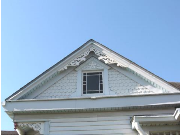
Anti-rot and anti-decay treatments like those described above can help with repairs if elements like bargeboard become damaged. (1013 W. Main Street)
