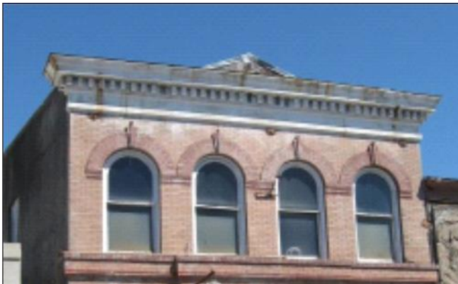
Upper façade detailing often includes sheet metal cornices such as at 1320 W. Main Street.
