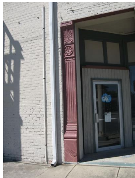
Cast iron features at 801 W. Main Street are important elements of 19th century commercial buildings.
