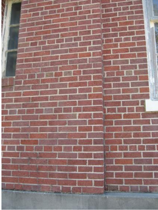
This brick exterior at 1614 W. Main Street is six-course common bond, having a header row every sixth course.
