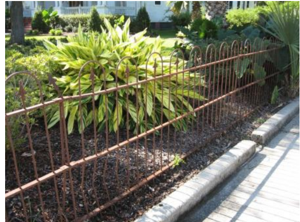
This original hoop and dart iron fence should be preserved. (1513 W. Main Street)
