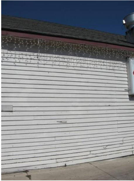
Original wood siding at 1400 W. Main Street
