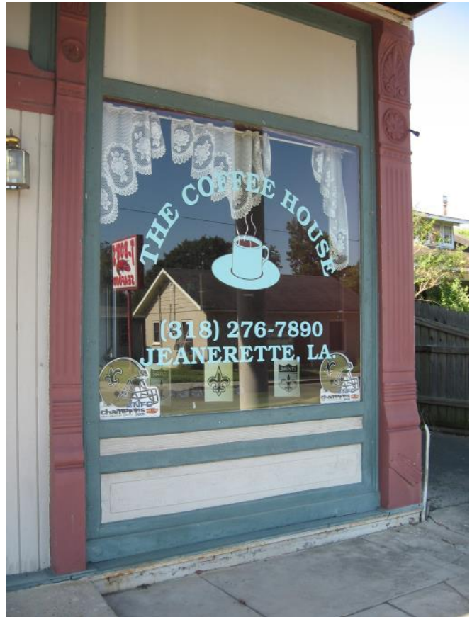
This historic storefront at 801 W. Main Street possesses many typical elements: original display windows, original frame bulkheads and cast iron pilasters. The transom has been enclosed and should be reopened in future rehabilitation.
