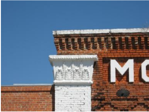
Corbelling and pilaster capital at the Moresi Foundry.
