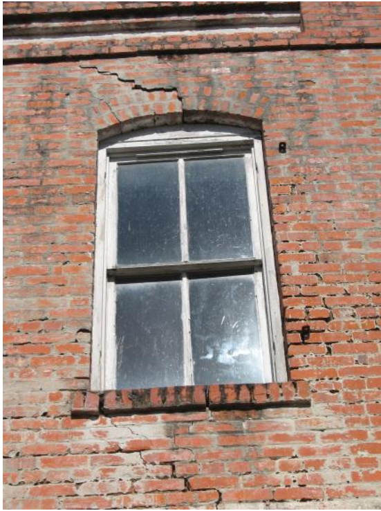
Original, two-over-two, wood sash window at 1503 W. Main Street.
