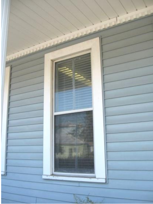
The design of this storm window, with a central meeting rail to match the historic window behind it is appropriate. (1440 W. Main Street)
