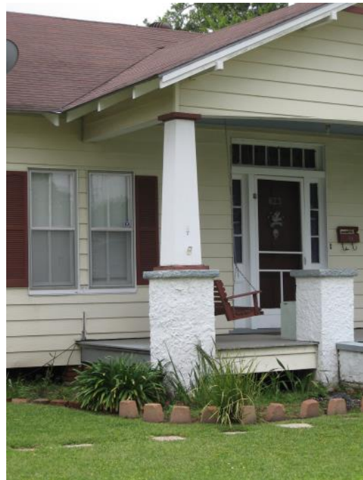
Porches on Bungalows such as this one at 632 W. Main Street often have tapered wood posts on masonry piers.
