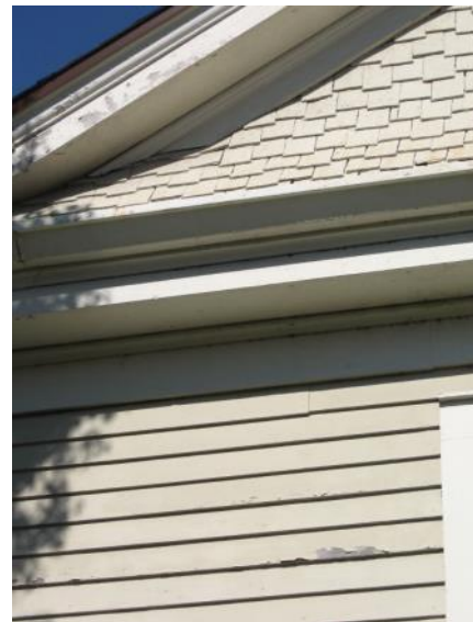
Wooden shingles help define the house's historic appearance. If they become damaged they should be repaired in accordance with the guidelines for wood. (1533 W. Main Street)
