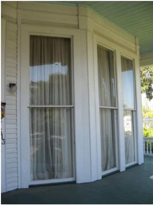
Original, one-over-one wood sash windows. (1513 W. Main Street)
