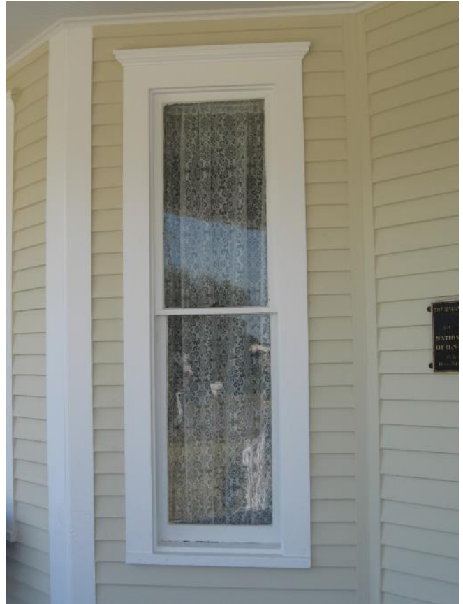
Original windows should not have original surrounds or cornices removed or concealed. (1617 W. Main Street)
