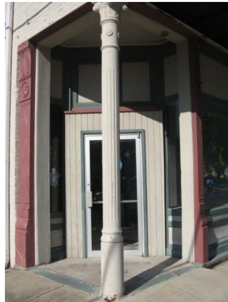
Cast iron columns, like this one at 801 W. Main Street were common features on 19th century and early 20th century commercial buildings.
